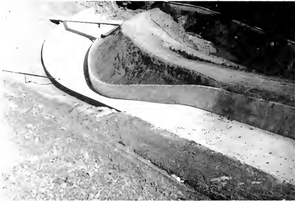
View of completed spillway extension
